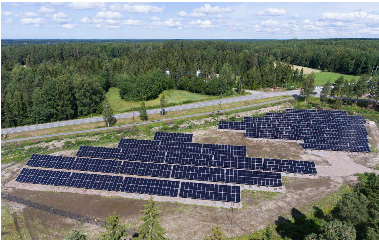
Solar park at Coreplast Laitila Oy.
