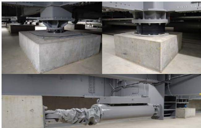
Hybrid seismic isolation structure
